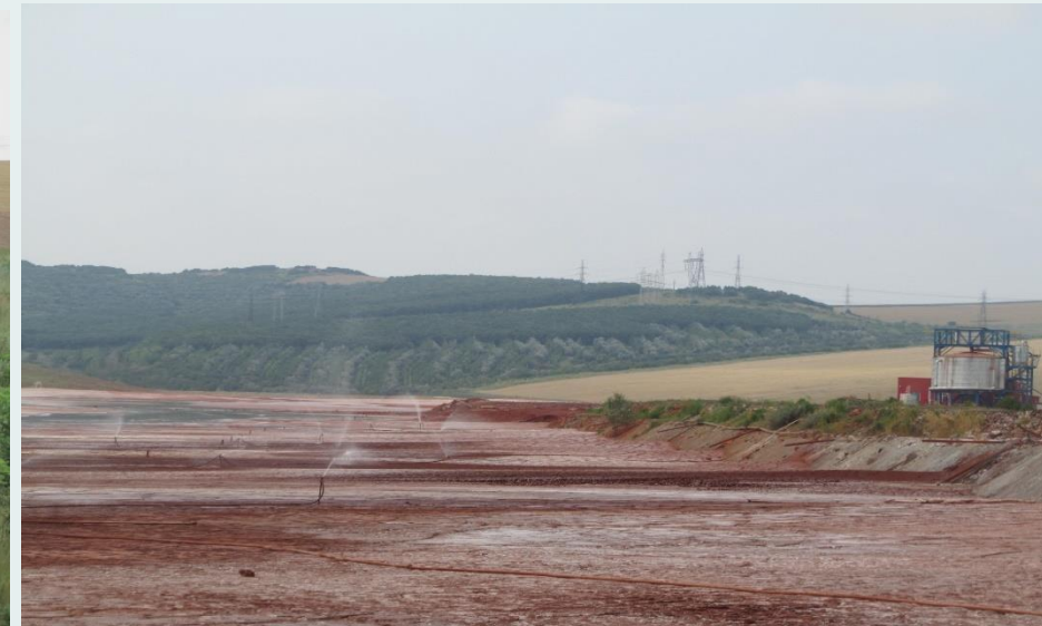
P6. Paste thickener & red mud moistening sprinklers
