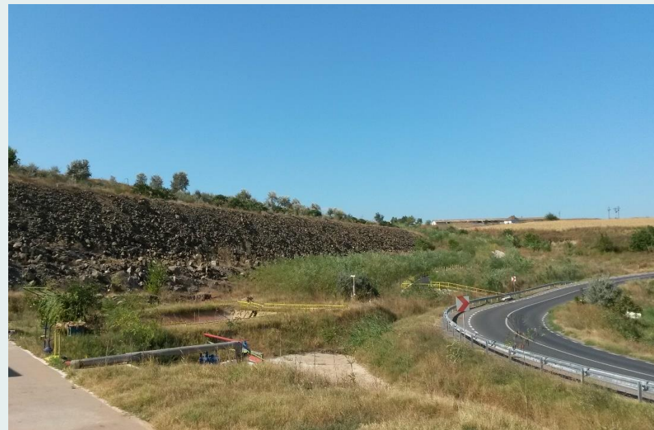
P1. Frontal dam, illuminated fencing and pumping station
