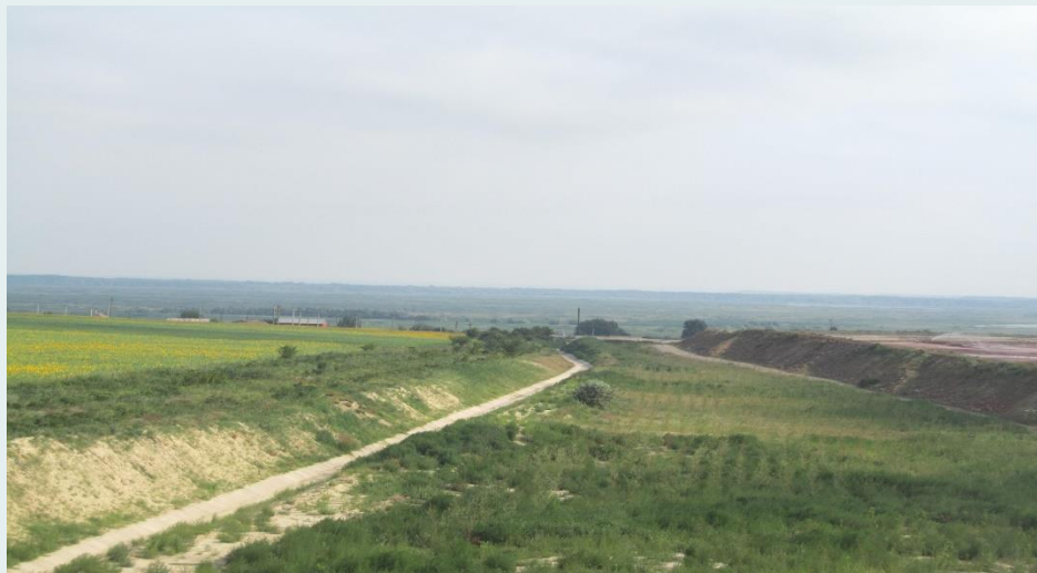
P3. Dyke and pluvial water detouring channel
