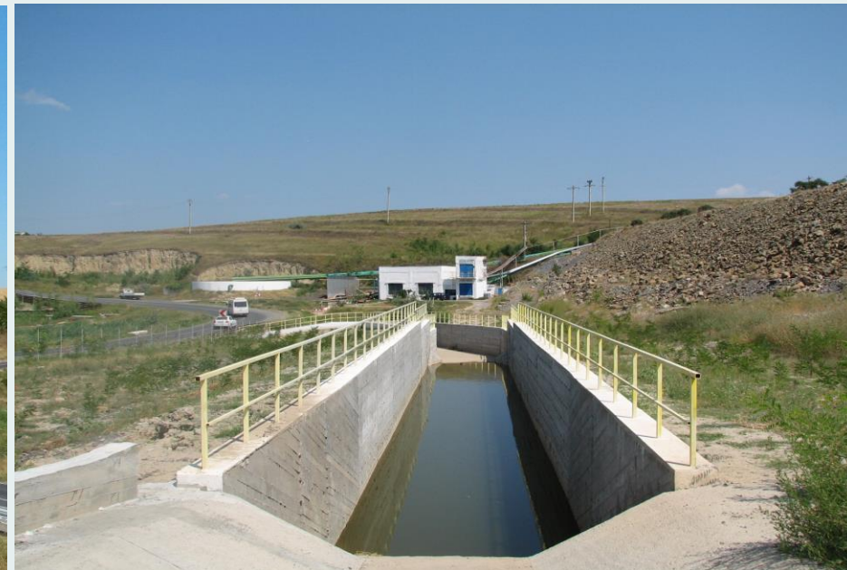
P2. The last part of the collecting pluvial water channel – designed to reduce speed of the rain water
